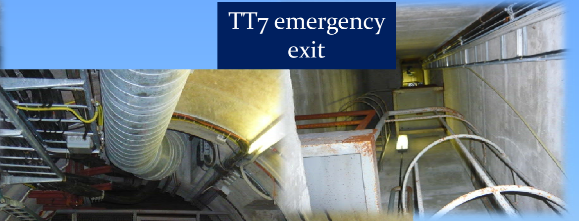
TT7 cable & ventilation shaft
